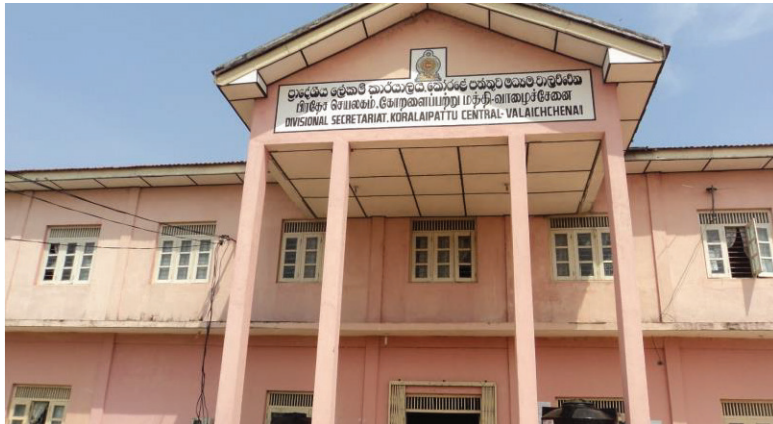
Figure 3: Koralai Pattu Central’s new divisional secretariat office
